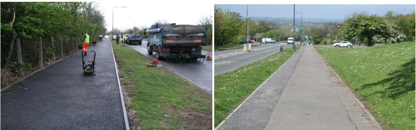
*(Pictures during construction and post construction of a 1.9 kilometre shared use path at Easthouses Road)*
