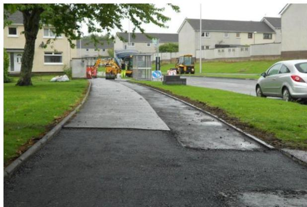
(Photos showing construction of “shared use” cycleway on Bogwood Road)
