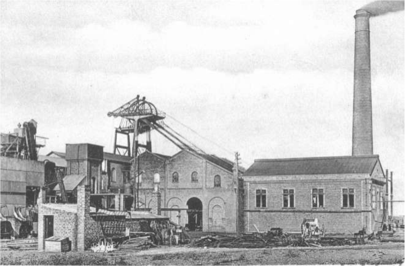
The Lady Victoria pit at Newtongrange was the centrepiece of the Midlothian coal industry. Owned by the Midlothian Coal Company, it was opened in 1895.
