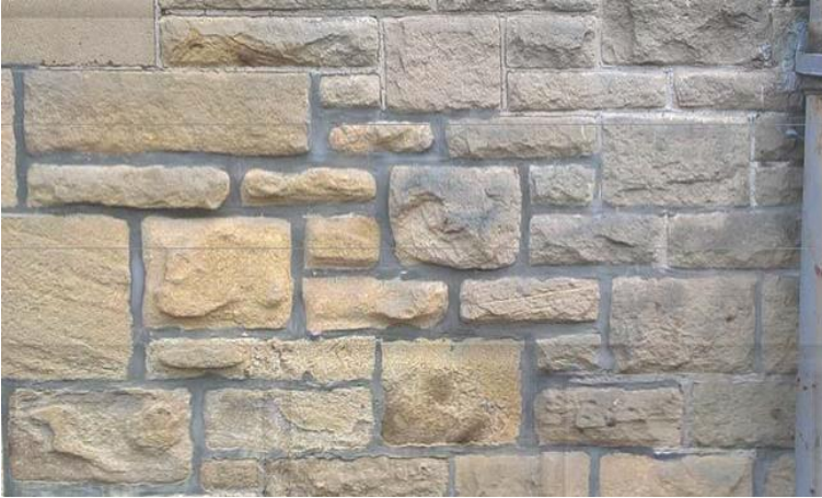
Evidence of recent cement pointing
