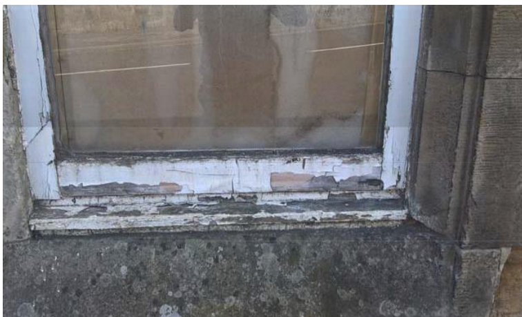
Evidence of lack of maintenance of paintwork on West Street
