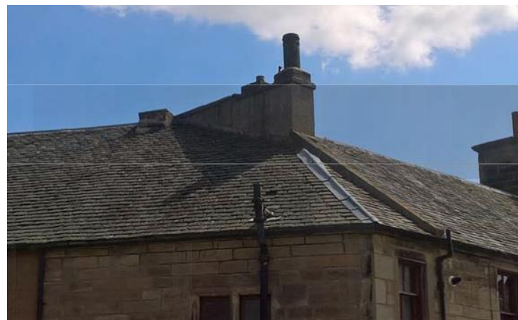
Truncated and cement harled masonry chimney stack
