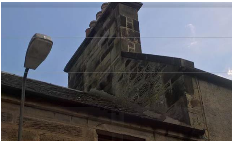
Failed cement fillet at base of gable and junction with slates
