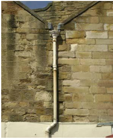
Water damage to masonry
