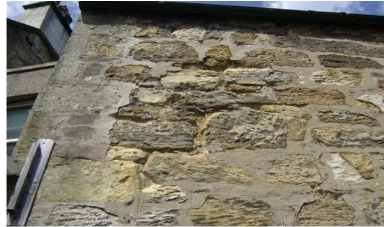
Cement over pointing causing rapid masonry erosion
