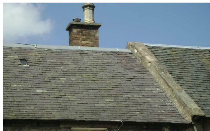
Welsh slate roof showing numerous patch repairs West Street
