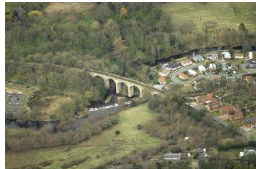
Lasswade Viaduct (aerial view)
