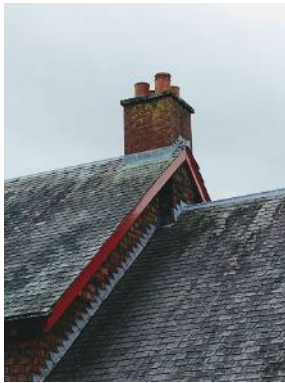
Chimney on cottage
