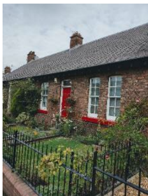
Single Storey Pit Cottage
