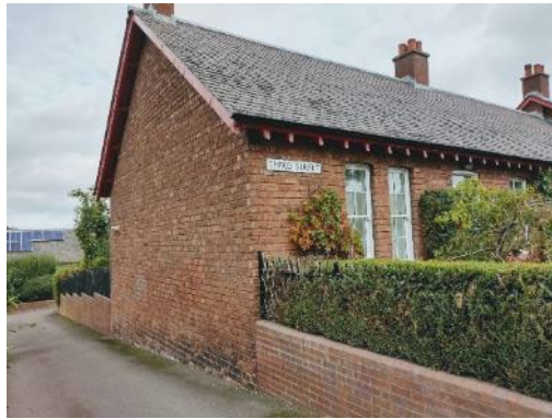
Exposed rafter ends
