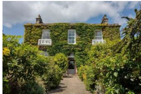
Door, windows and ironwork
