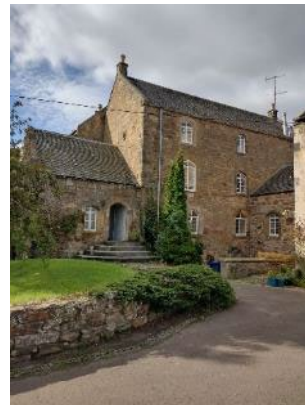
Former Ironmills mill buildings
