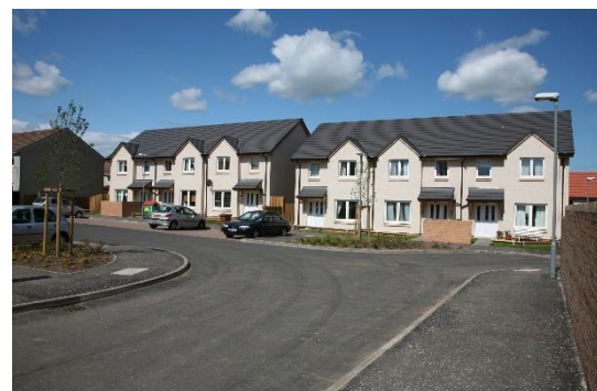
Figure 2: Midlothian Council housing in Bonnyrigg
