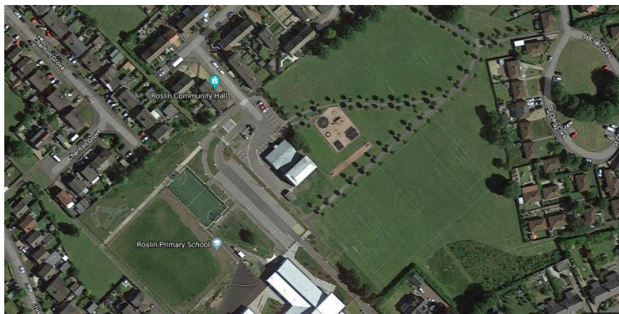
Figure 1.1: Aerial view of the Roslin Pavilion.
