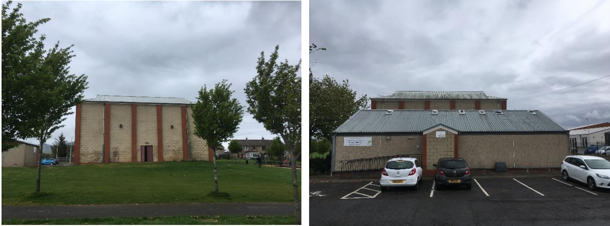
Figure 2.1: Front and rear photos of Roslin Pavilion.
