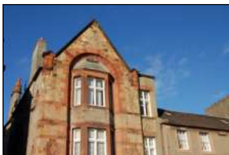
Dominant gable at Nos 37-39
