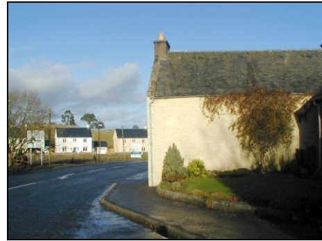
Gable end of No13 at right angles to the road forming an important visual stop.
