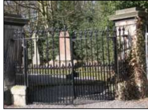
Squared stone gate piers with cast-iron fleur-de-lis ornamental railings
