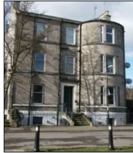
The former bank
