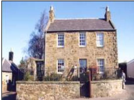
23 Main Street, a key building in the street scene is constructed of coursed-tooled rubble with ashlar quoins on the right corner and sandstone cills.
