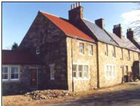
Sensitive refurbishment of dwellinghouse in Hill Road. Pantiles provide a hint of warmth to the street scene. Stone chimney stacks remain with their pots *in situ*.
