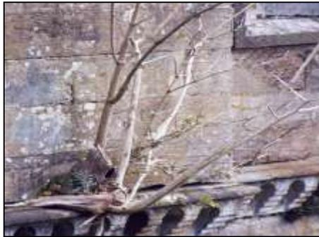
Damage caused by natural vegetation to Oxenfoord Viaduct.
