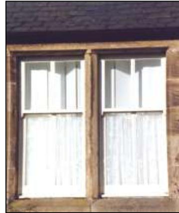
Vertical window opening with central stone mullion, bipartite sash window and chamfered arrises.
