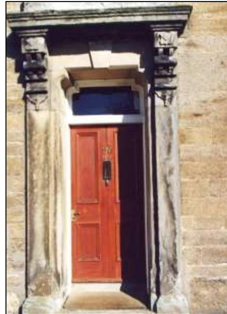
Elaborate stone detailed porch with splayed stone pilasters & ornamental carved bracket heads supporting the stone canopy.
